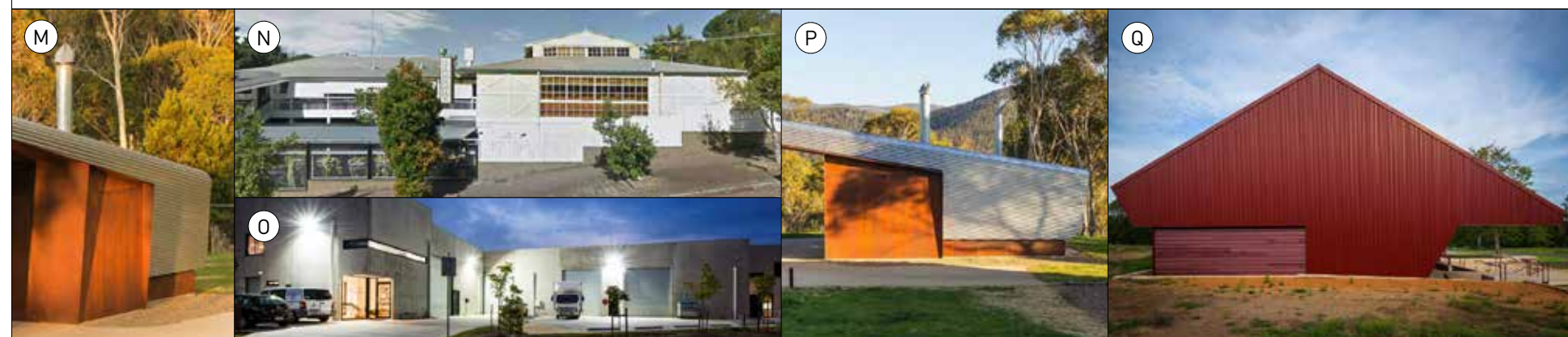
EXEMPLARS IMAGE: M & P, Vernacular materials - Profilled metal cladding; N, Eumundi Brewery Single skin walls; O, Precast Concrete walls - The gateway Noosaville; Q, Vernacular materials - Profilled metal cladding & weatherboard - Toogoolawah Dairy
