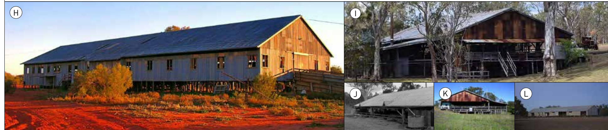
SCALE CONTEXT IMAGE: H, Outback Shearing Shed; I, J & K, Elgin vale Sawmill; L, Cordillo Downs Shearing Shed
